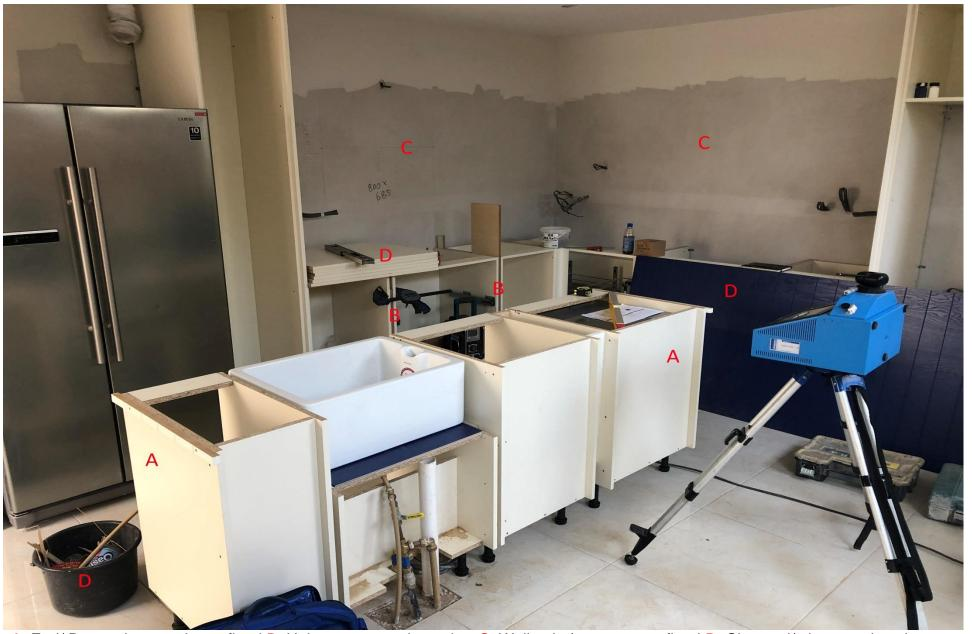
A: End/ Decorative panels not fitted B: Units not secured together C: Wall units/extractor not fitted D: Cluttered/ obstructed work area More examples at <a href="https://drive.google.com/open?id=1APwNxLpOou9eRMMsoX3nQ8h-2WGVY2V9">https://drive.google.com/open?id=1APwNxLpOou9eRMMsoX3nQ8h-2WGVY2V9</a>
