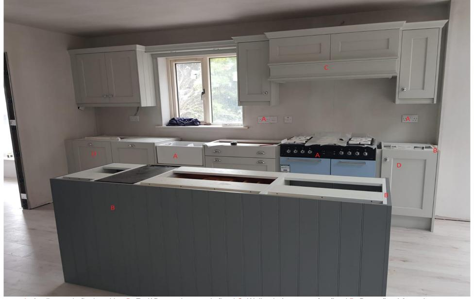
A: Appliances in final position B: End/ Decorative panels fitted C: Wall units/ extractor fan fitted D: Doors fitted & on site. More examples at <a href="https://drive.google.com/open?id=11v5mqozRkPRc3JgbYt-yemEDAF4Ww">https://drive.google.com/open?id=11v5mqozRkPRc3JgbYt-yemEDAF4Ww</a> Ye
